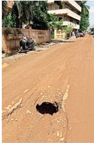
A gaping hole has appeared on the Idgah Road in Varthur
