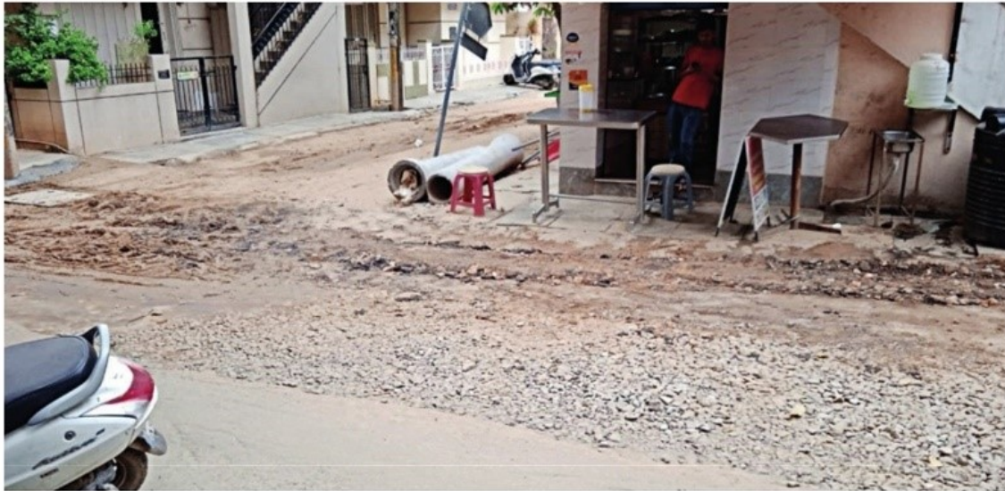
The stretch is unpaved, making it unsafe for walking and driving
